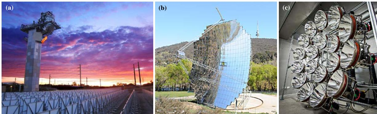
Figure 1. Flagship Australian CST research facilities: (a) 1MW<sub>th</sub> solar tower at CSIRO, (b) 0.5 MW<sub>th</sub> Big Dish at ANU, and (c) 45 kW<sub>e</sub> high-flux solar simulator at ANU.
