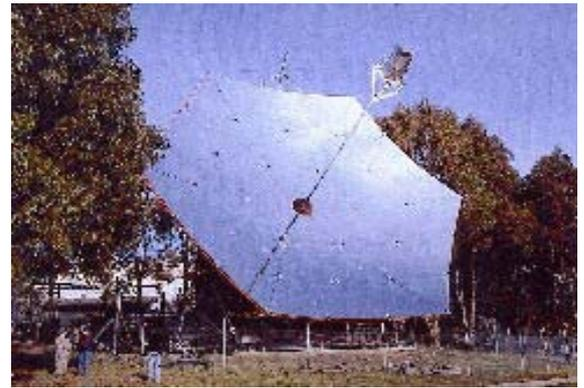
Figure 1: ANU's 400m<sup>2</sup> Paraboloidal Dish
