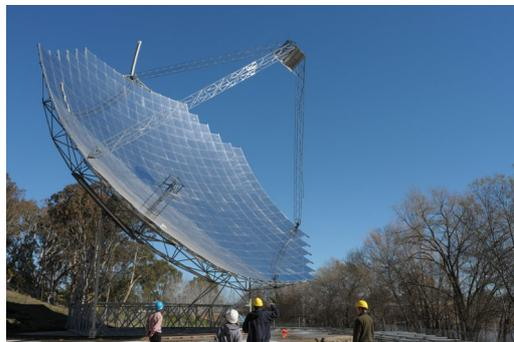
**Fig. 1. SG4 parabolic dish, with a surface made from 380 mirror panels.**
