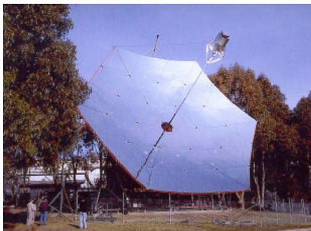
Figure 1: 50 kW<sub>e</sub> prototype solar power plant using ANU's 400 m<sup>2</sup> paraboloidal dish.
