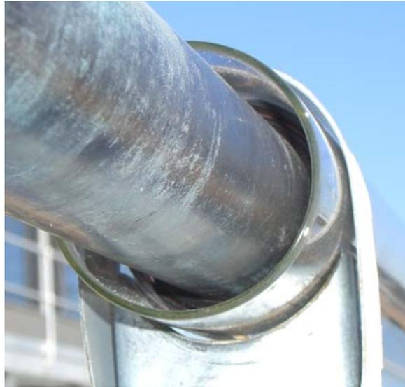
**Figure 2.5 View of absorber tube inside glass tube**
