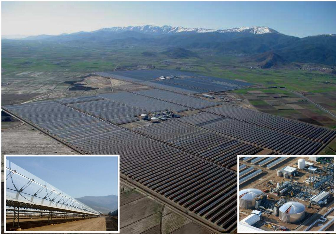
Fig. 1: An aerial view of the Andasol-1 and Andasol-2 plants (Photo: Protermosolar). *Left inset:* Parabolic troughs tracking the sun at Andasol-1 (Photo: Author). *Right inset:* The hot and cold salt tanks and power block during construction (Photo: Protermosolar).
