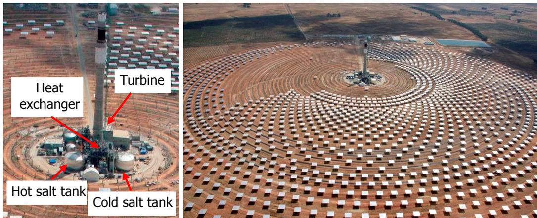
Fig. 6: Construction of the Torresol Gemasolar molten salt power tower
