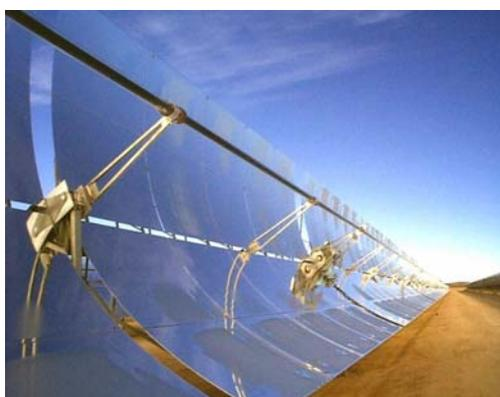
**Figure 1—2 : An array of LS-2 trough concentrators in California.**
