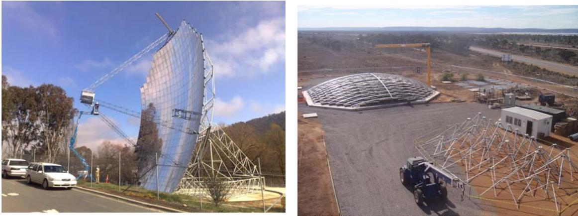
**Fig. 2. The “SG4” Big Dish prototype on campus at the Australian National University (left, Aug 2009) and early construction work of Big Dishes in Whyalla (right, May 2010).**
