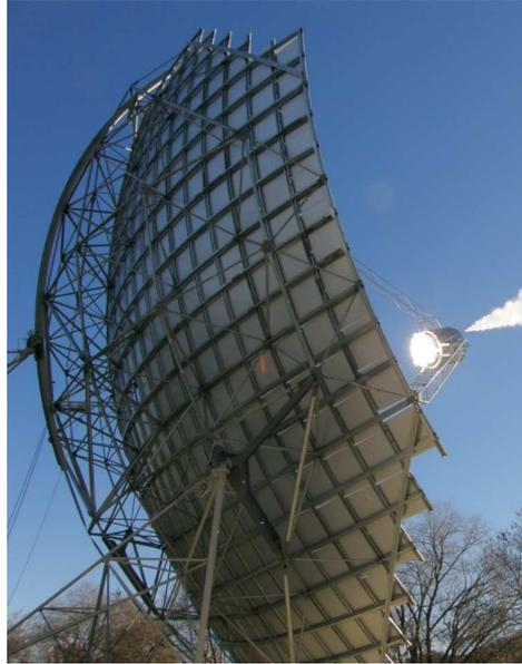
**Fig. 1: Rear view of SG4 dish, showing space frame structure and square mirror facets.**
